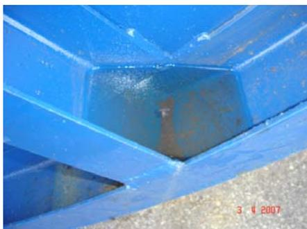
**Figure 3. Central axle holding water**
